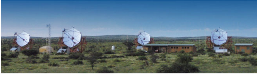
Fig. 25. Photograph of the four H.E.S.S. 12-m diameter Cherenkov telescopes in the Khomas Highland of Namibia. The future 28-m diameter H.E.S.S. II telescope will be located in the center of the four telescopes.
