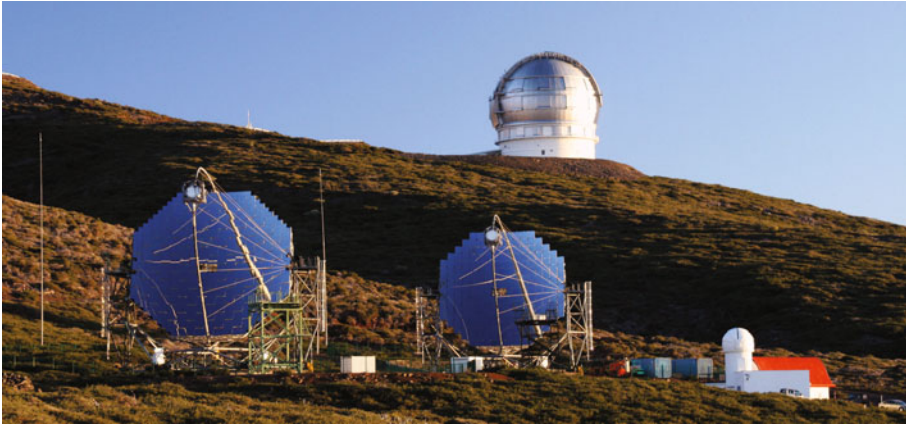
Fig. 27. Photograph of the two 17-m diameter MAGIC telescopes on La Palma. The two MAGIC telescopes are located in the foreground, 85 m from each other. The red-roofed house is the control house. In the background the 10-m optical Gran Telescopio Canarias as well as the 2.5-m Nordic Optical Telescope (upper left) are visible.
